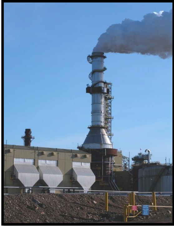
UE-1 Expansion Plant Alberta, Canada
