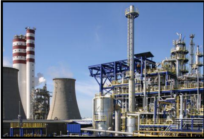
Combined Heating and Power Plant | Pulawy, Poland
